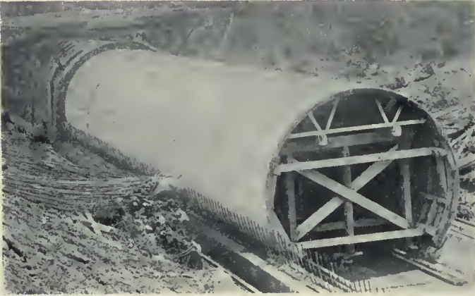
Inner form in place, outer form and pouring platform in background.
